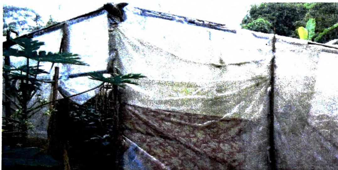
A Substandard Structure Covered with Old Sarees
