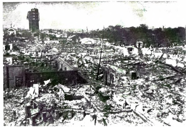
Collapsed 13 story masonry wall tower after Kanto Great Earthquake 1923
