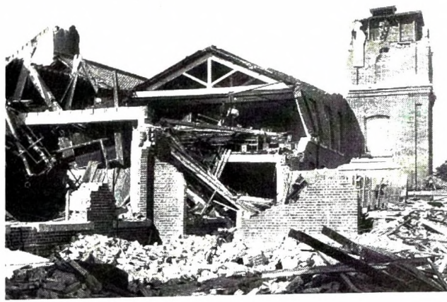
Damaged brick factory constructed by imported technology after Nobi Earthquake 1891
