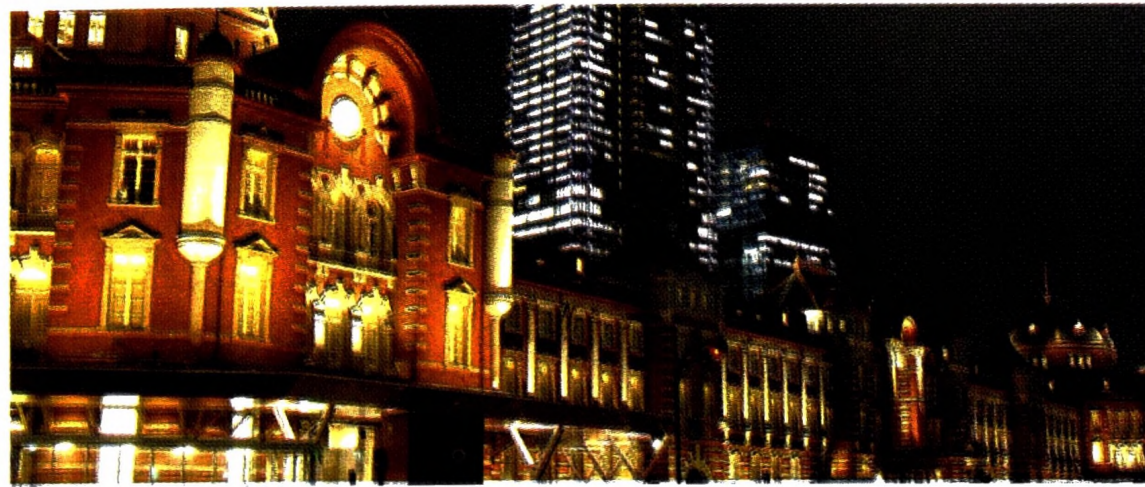
The Tokyo Station constructed in 1911 and completed retrofitting by seismic isolation on 2010.
