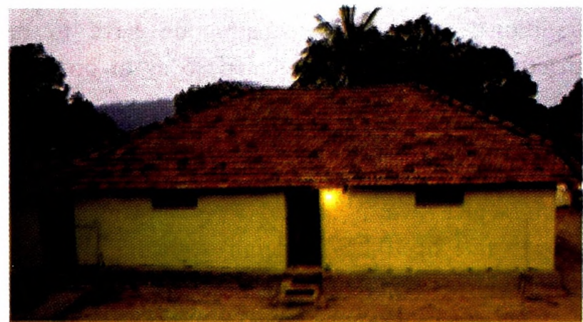
Fig.15. Hut at Coorg modified with tile roof
