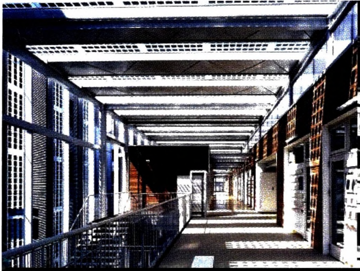
Fig.23. Solar Curtain Wall Type for Daito Bunka University
