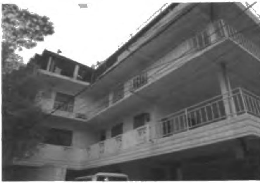
Figure 01: A four story Building (12 Apartments)
