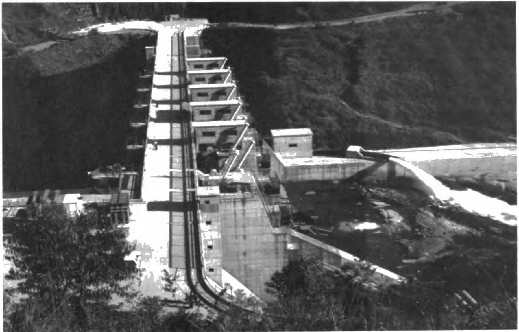
Aerial View of the Upper Kotmale Hydro Power Project Dam
