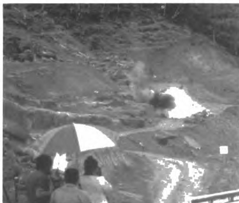
Ceremonial First Blast at Power Cavern on April 9,2007
