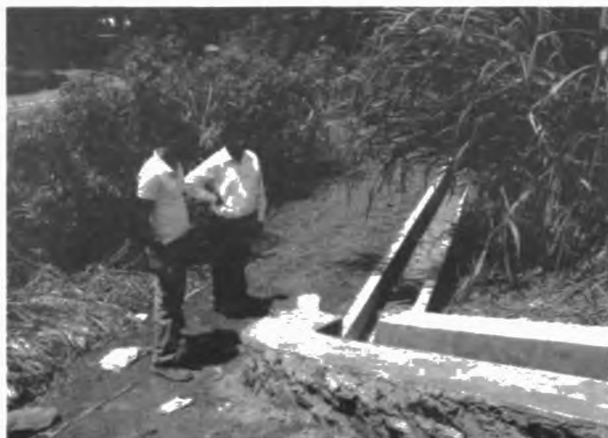
Figure 13 - Construction of a Drainage System at Sumana Maha Vidyalaya Talawakelle
