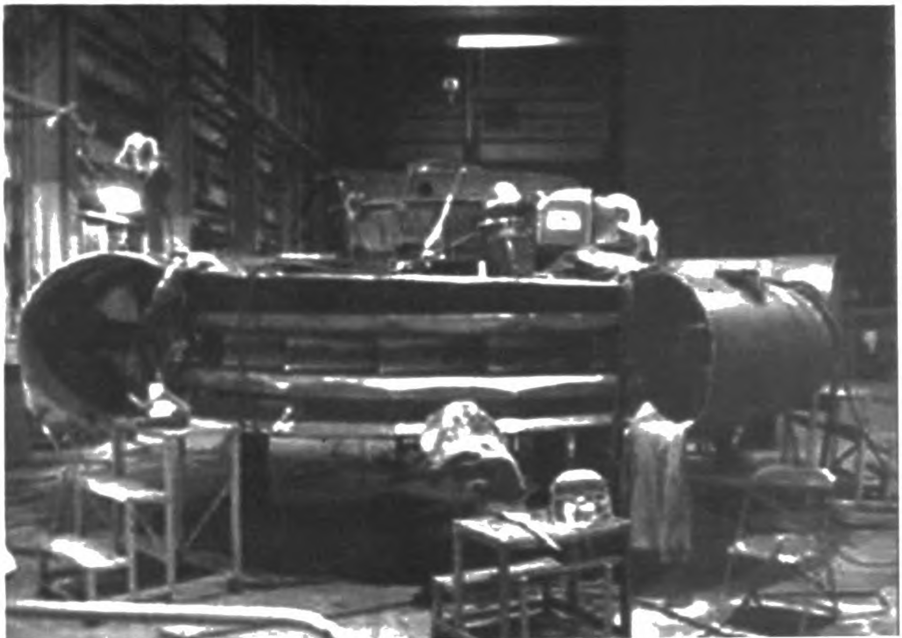
Spiral Casing of the Turbine
