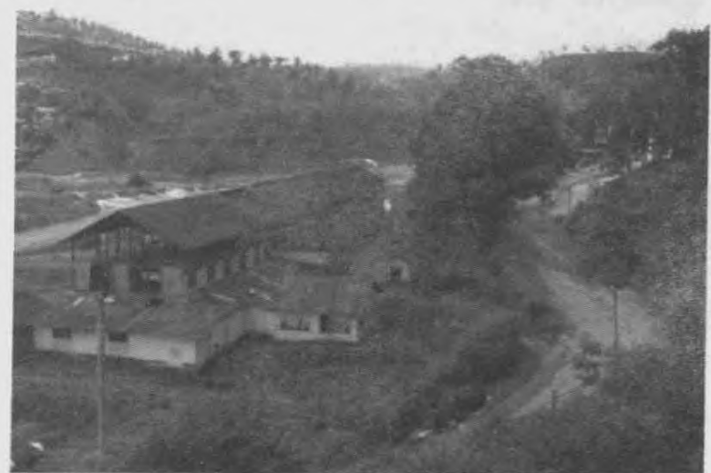
Figure 14 - Old Tamil School Building after shifting being vandalised
