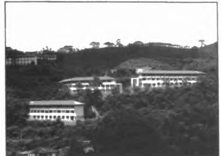
Figure 18 - Buildings Constructed for Tamil Maha Vidyalaya
