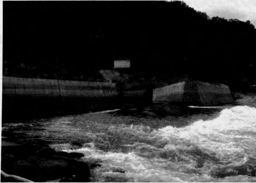
Figure 12 - Photograph of the Outlet
