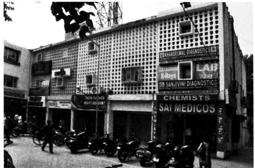
Fig8: Sector -11 market is now most happening place with variety ofshops/ activity. (Source: Rajiv,ccaPhotographer)
