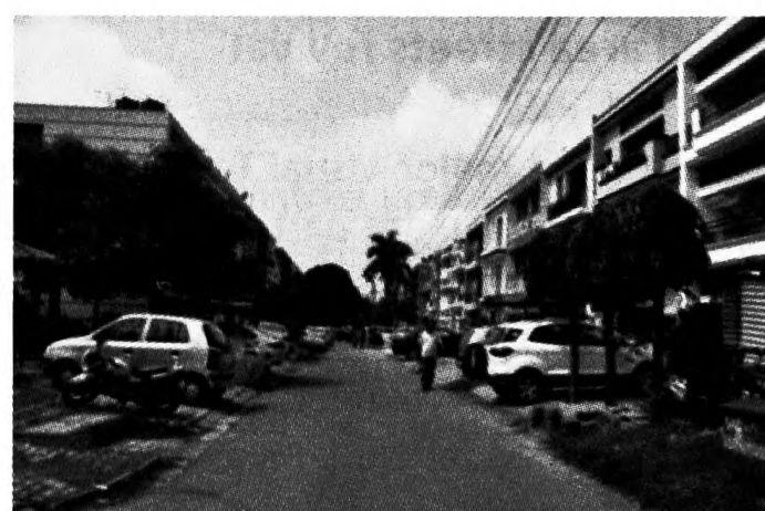
Fig10: Parking problem already visible on Marla houses street in sec-46 (source: Rajiv, CCA)
