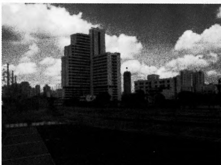
Fig. 6: A View of Klong Phai Singh To Source: The Crown Property Bureau
