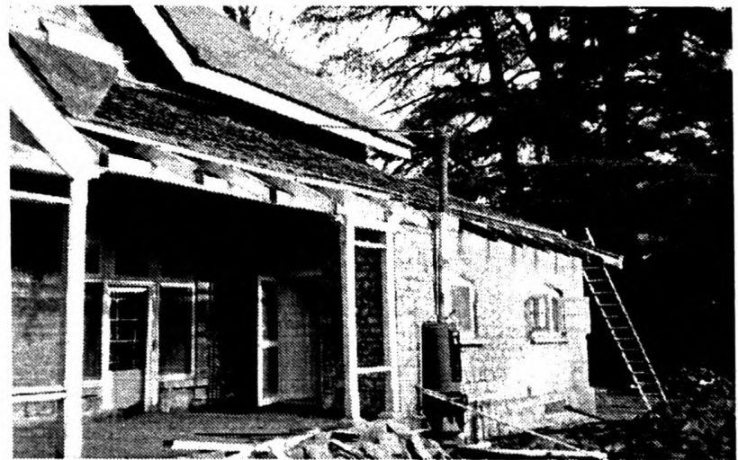
Fig. 4: Frontier House Back Side View Source: Author
