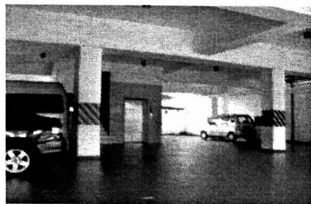
Fig 27 - Car park is dominant all over ground floor in both case 02 and 03 Source - Author
