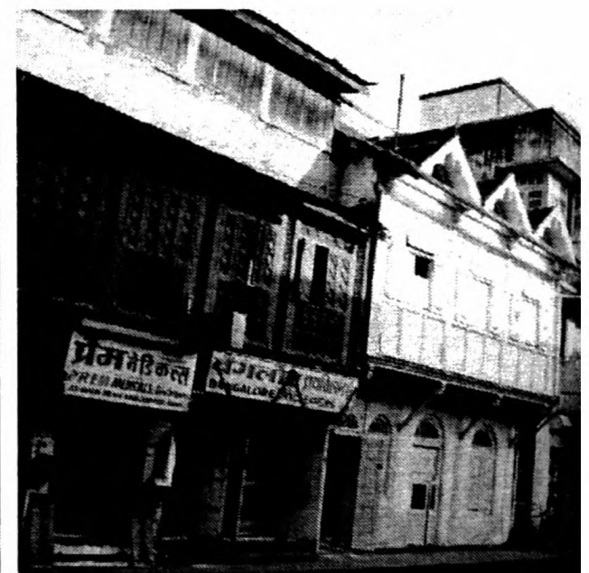
Fig. 27: Structure on D M Road, Source: The Author
