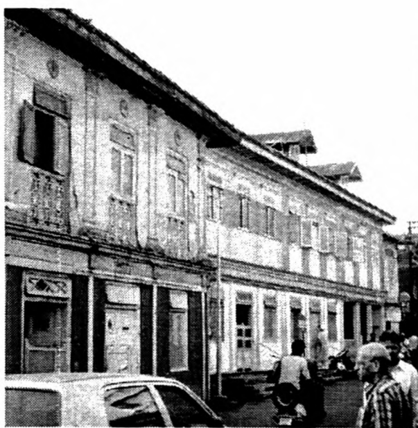
Fig. 25: Structure on D M Road Source: The Author
