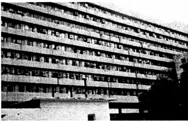
Fig. 6: A typical office building Source: The Author
