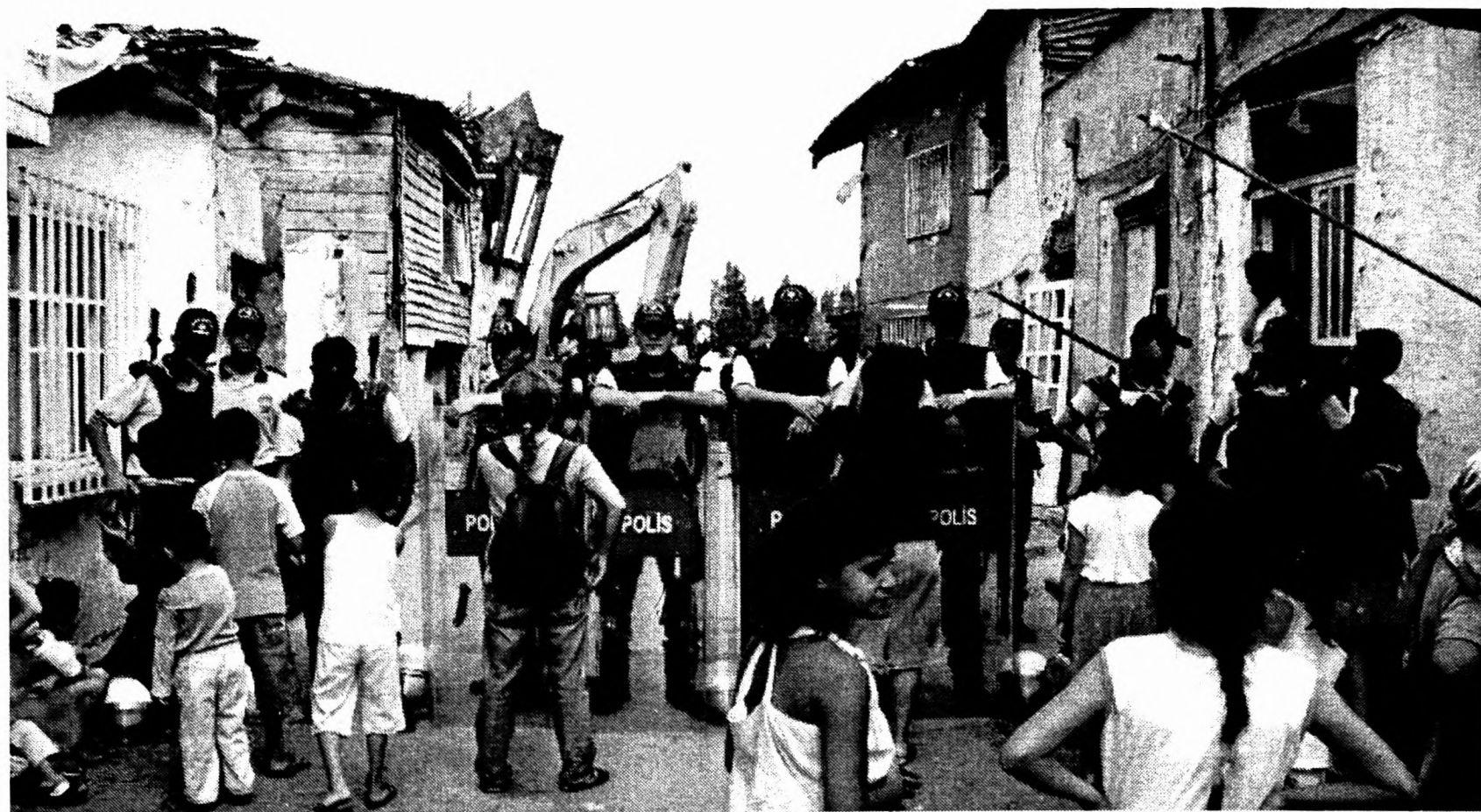
Fig. 12: Demolishing day in the neighbourhood, 2008 Source: http://sulukulegunlugu.blogspot.com/
