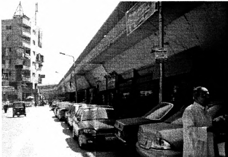
Fig. 7: Shops beneath Faysal Bridge Source: author
