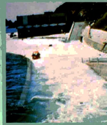
Oga Aquarium, Akita Japan. Parking lot of aquarium is flooded stranding car during the May 26, 1983, Japan Sea tsunami. (Takaaki Uda, Public Works Research Institute, Japan)
