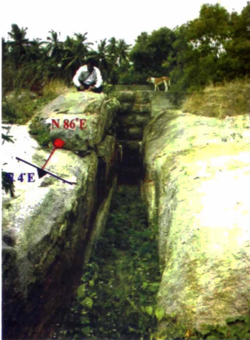
Fig. 4 Water diversion through the jointed rock mass at the abutment of the tank bund.
