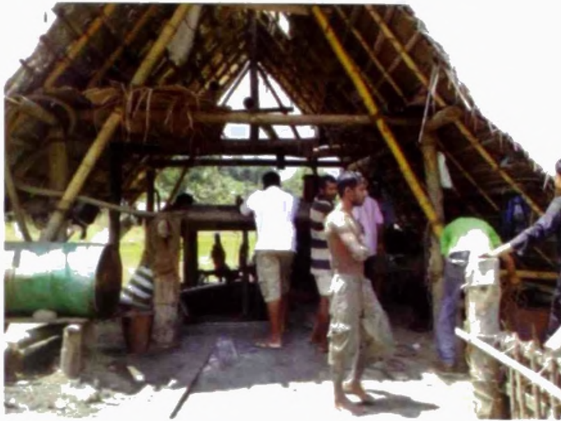
Plate 1 Shed built using bamboo trees, arecanut trees, and coconut leaves to protect the gem mine from rain, Braod valley at Pelmadulla
