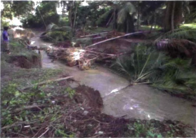
Plate 1 Newly built channel after meander cutoff.
