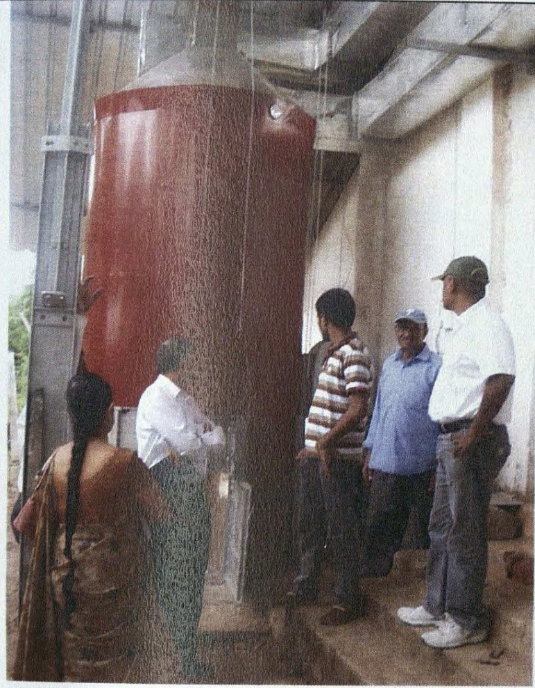
Figure 1: Hot air generator
