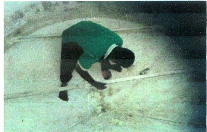
Cleaning of bottom of conical shape tank
