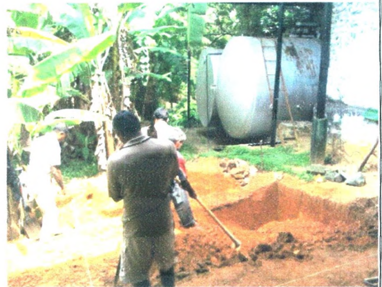
Foundation work started
