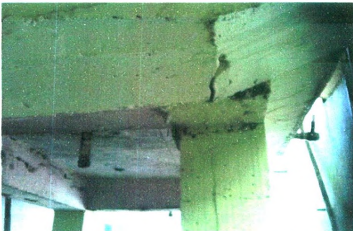
Washout of the rectangular tank
