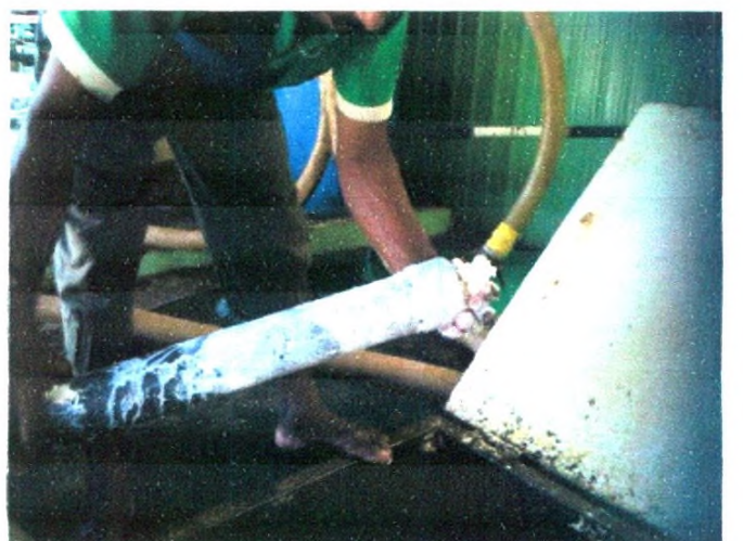
Cleaning of clogged valve
