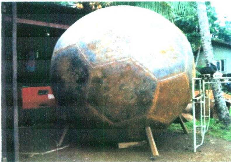
22500 liter Mild Steel Spherical Tank
