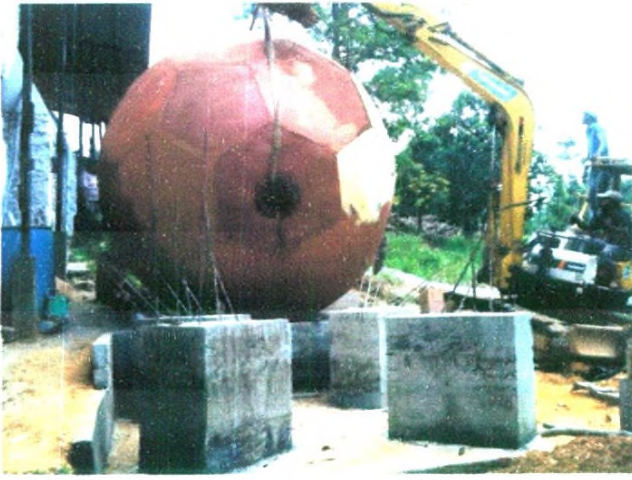
Positioned on the base foundation
