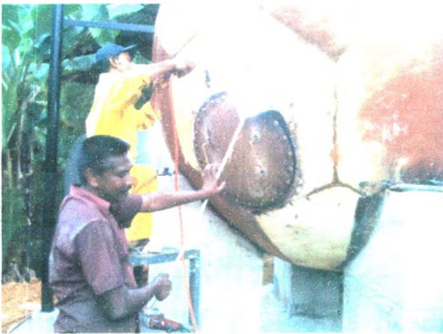
Fabricated the side manhole
