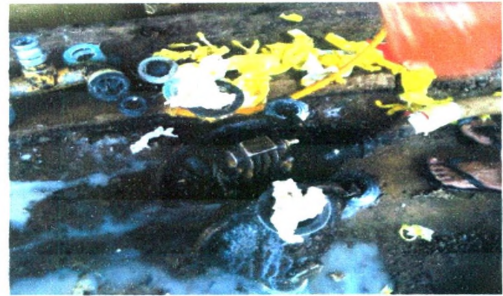
Dismantled vacuum pump due to clogging
