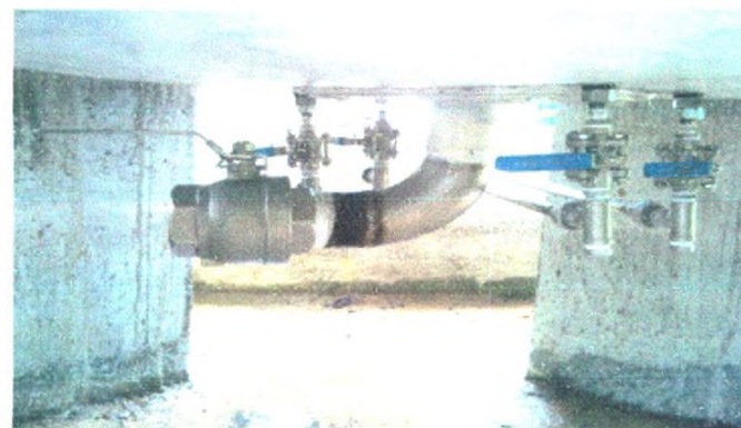
S/Steel nozzle assembly with outlet pipe
