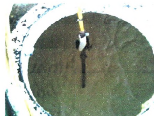
Ammonia gas supply lines to centrifuged latex maturation tanks
