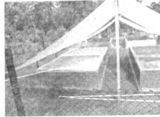
Tank Covered with mosquito Netting to prevent insects falling in
